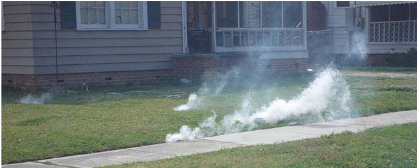
Smoke testing verifies leaks in sewer lateral pipes
